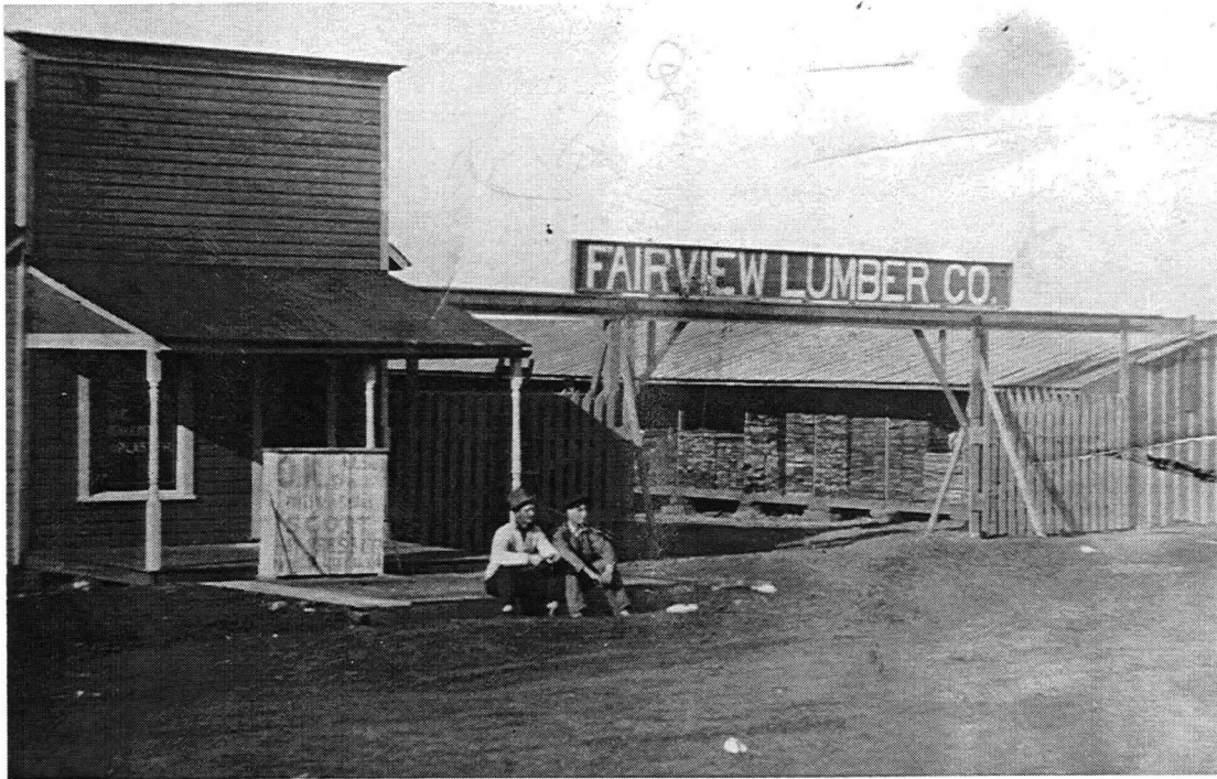
Louis Plumer managed lumber yards in Lucien, OK from 1908 to 1917, through a succession of ownership changes. Here he is, seated at right, in front of the Fairview Lumber Yard about 1911.
